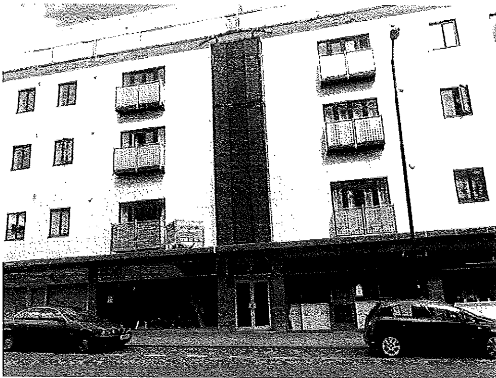
Flats immediately over the proposed night club with balconies and windows
